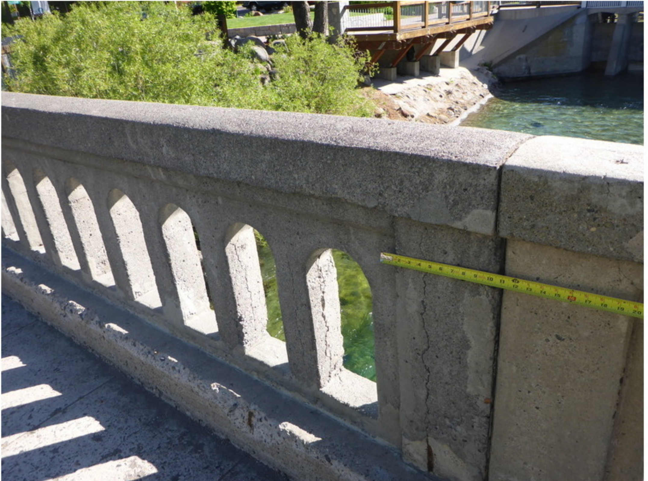
Photo No. 2 Ballusters With Incipient Spalling (typ)
