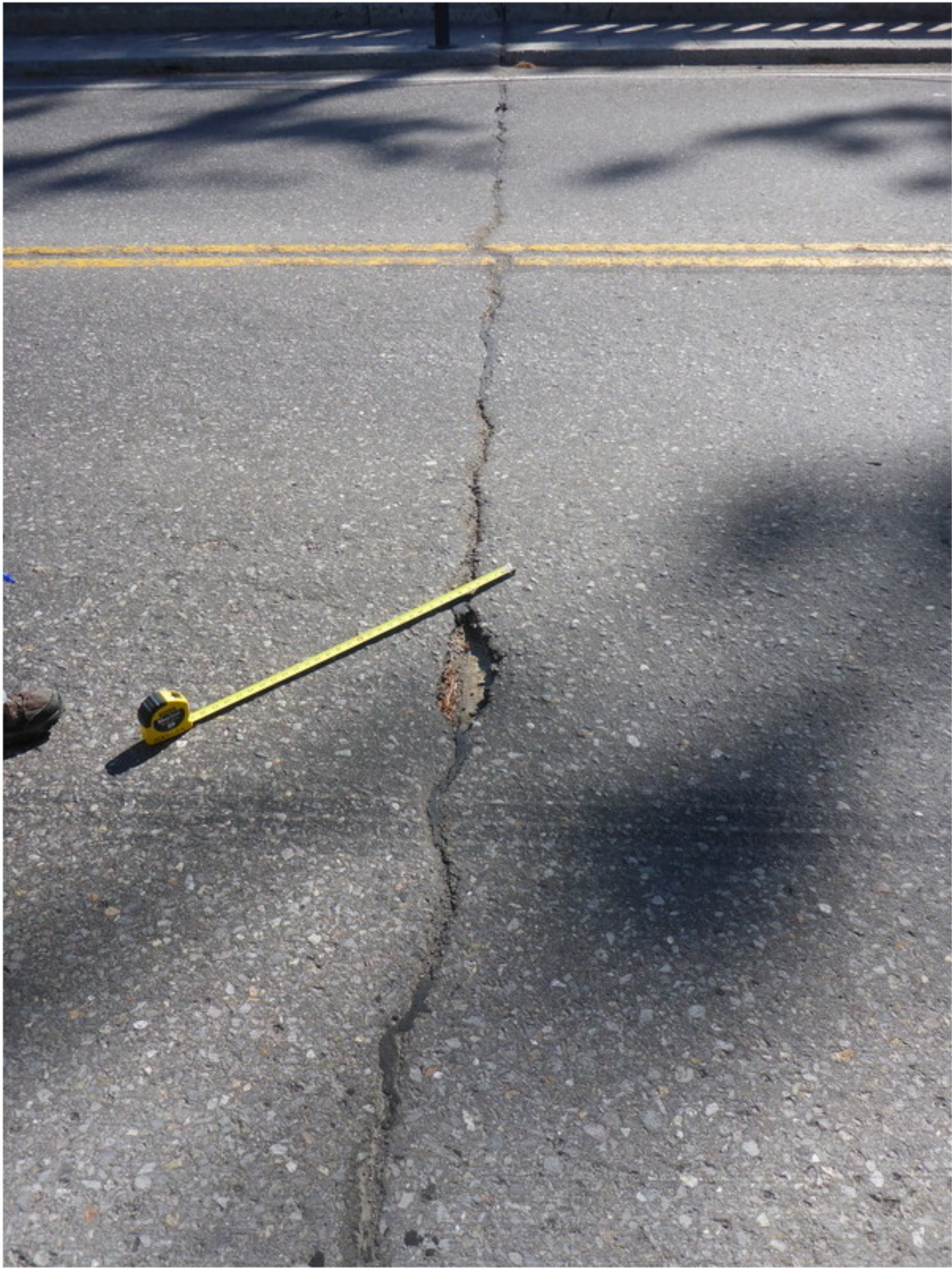
Photo No. 6 Transverse AC Cracks, Abutment 1 Joint
