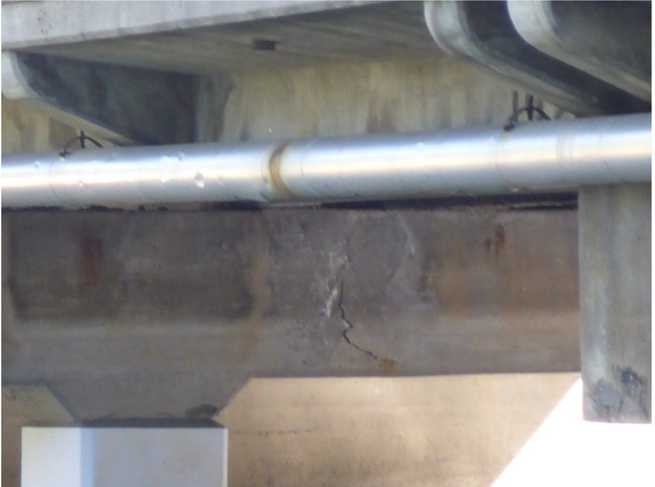
Photo No. 9 Bent 2 Cap Left Side Overhang: Incipient Spall
