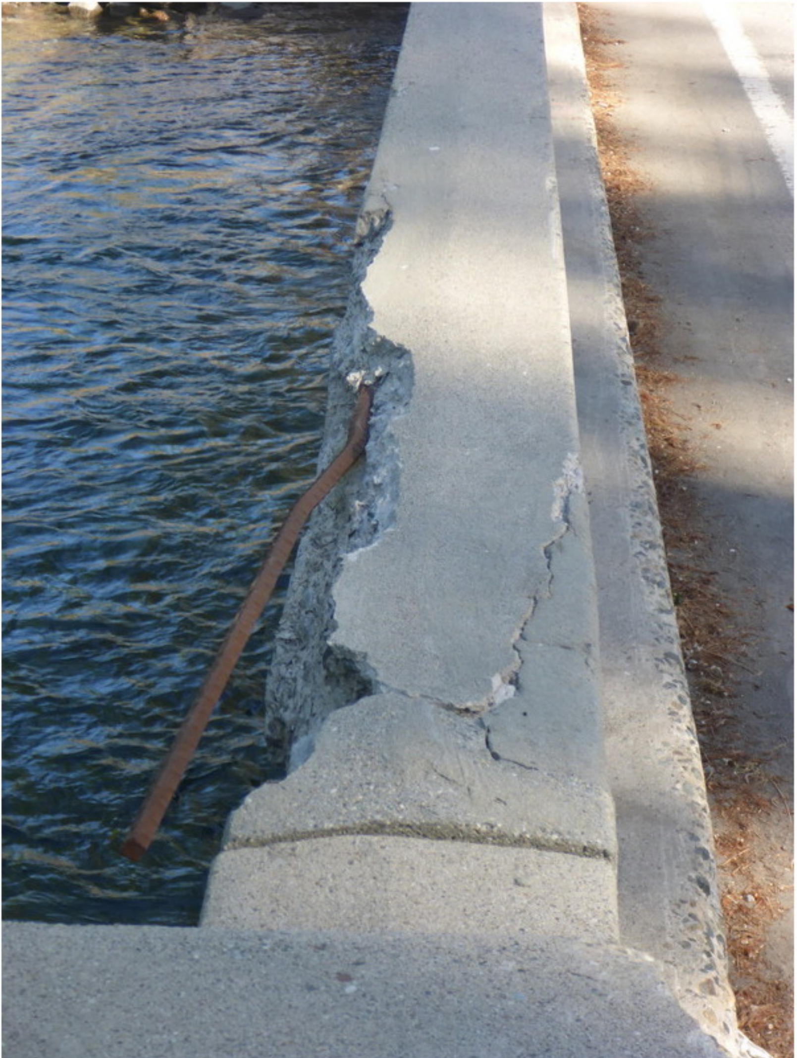
Photo No. 3 Spalled Rail With Exposed Reinforcement Near Abutment 1 (Left Side)
