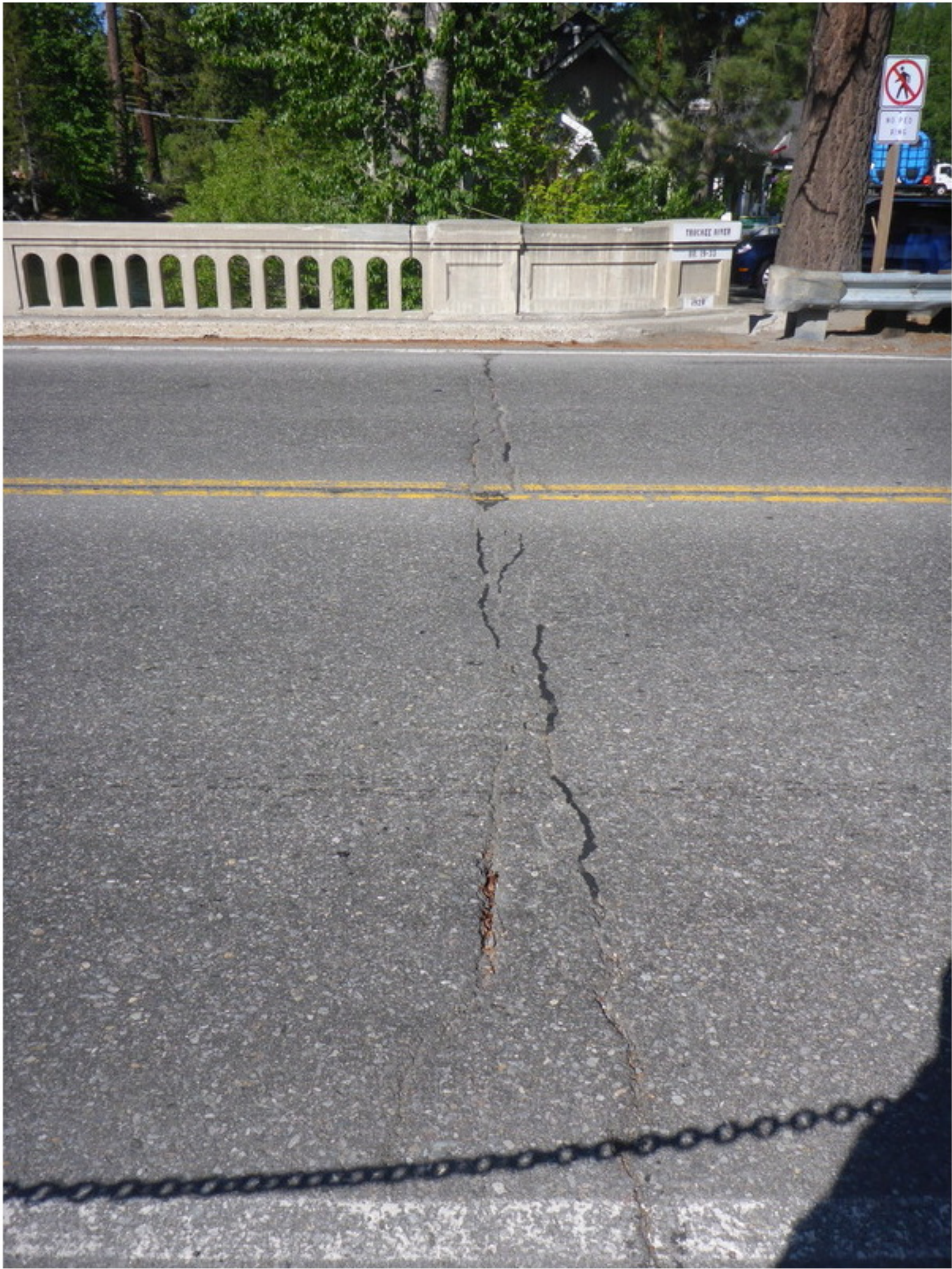
Photo No. 5 Transverse AC Cracks, Abutment 5 Joint
