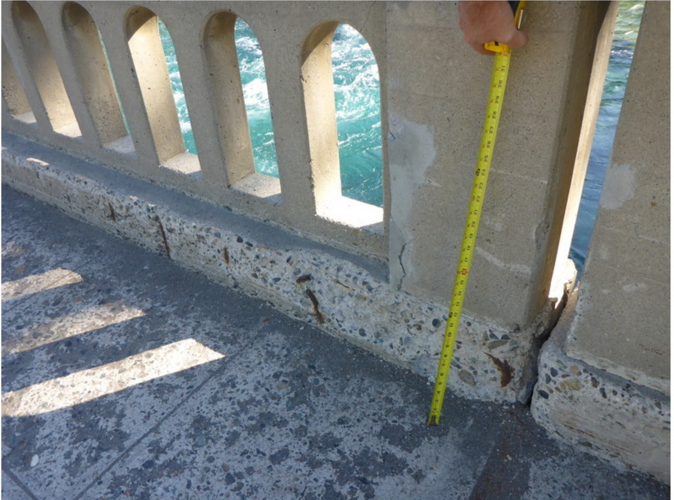
Photo No. 1 Spalled Rail Base With Exposed Reinforcement (typ)
