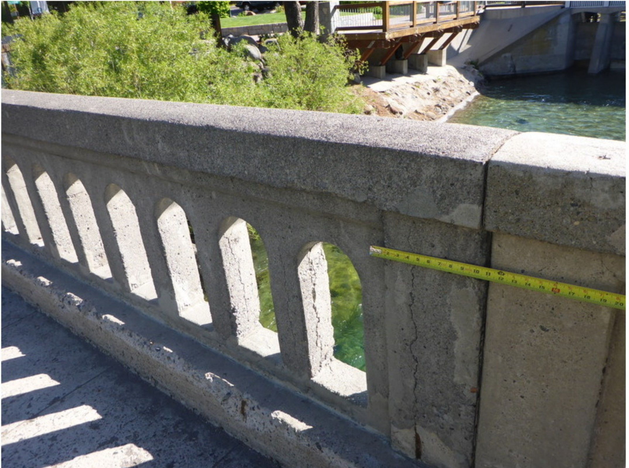
Photo No. 2 Ballusters With Incipient Spalling (typ)
