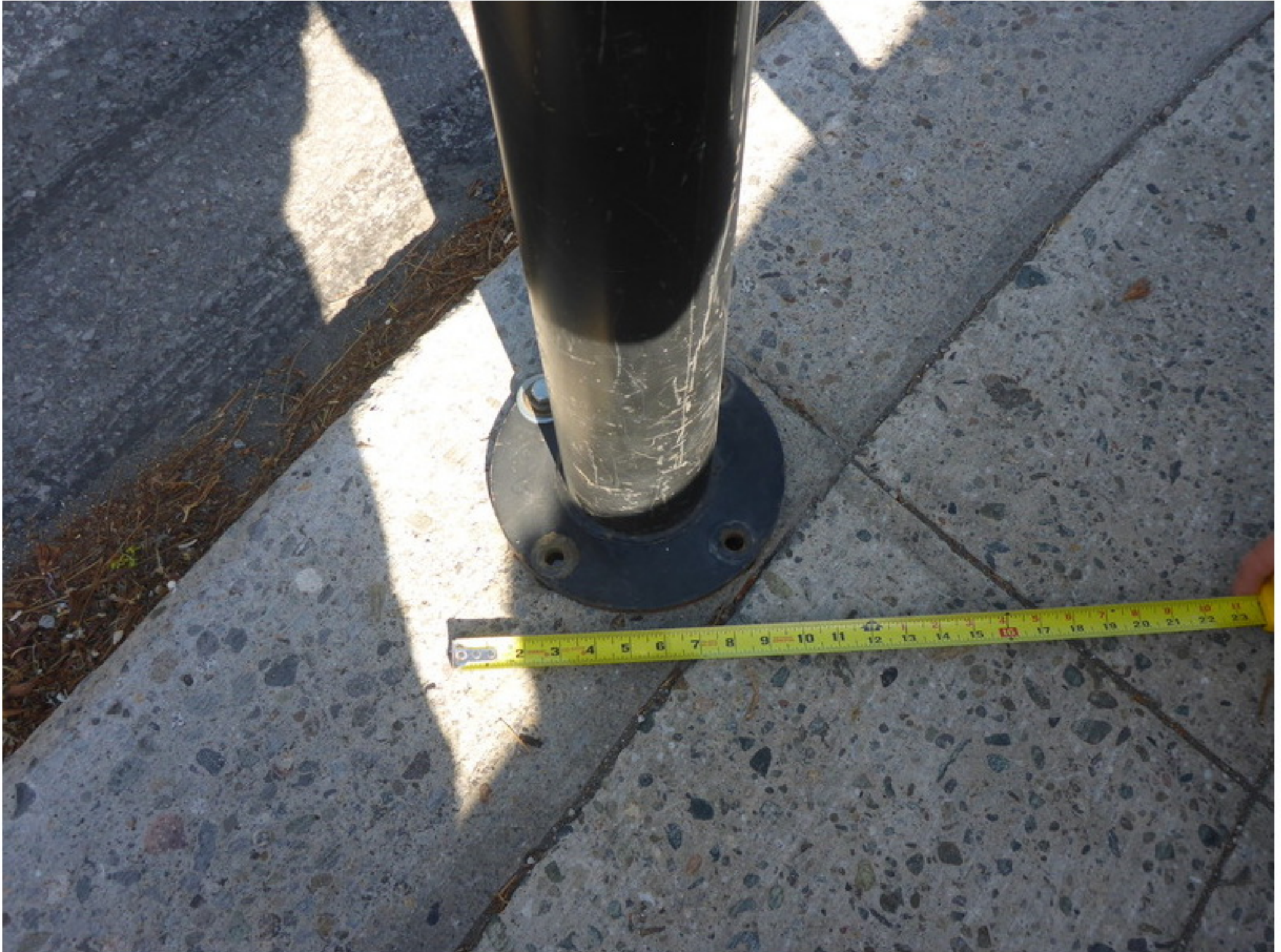
Photo No. 4 Railing Stanchion With Missing Bolts (typ)
