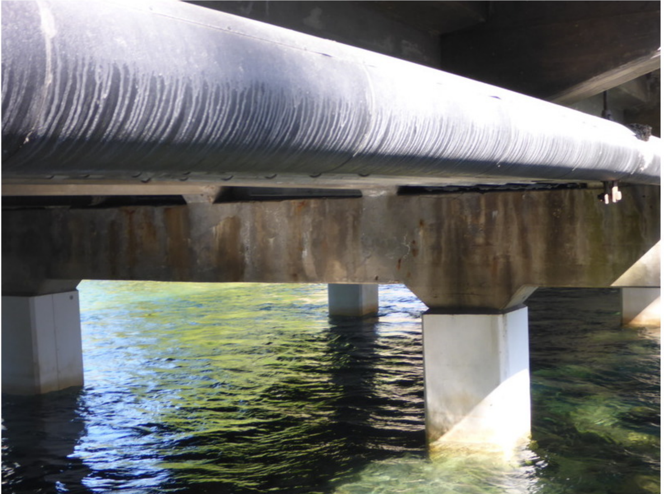
Photo No. 8 Bent 2 Cap: Patches, Map Cracking, Efflorescence and Staining
