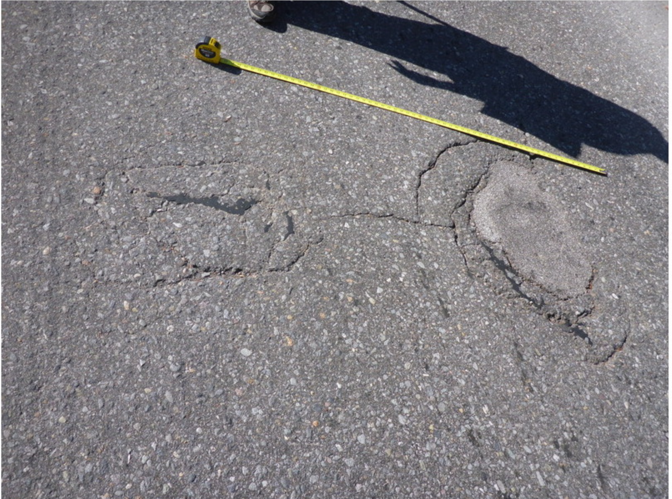
Photo No. 7 Failed AC Section with Patch, Span 3 Left Side
